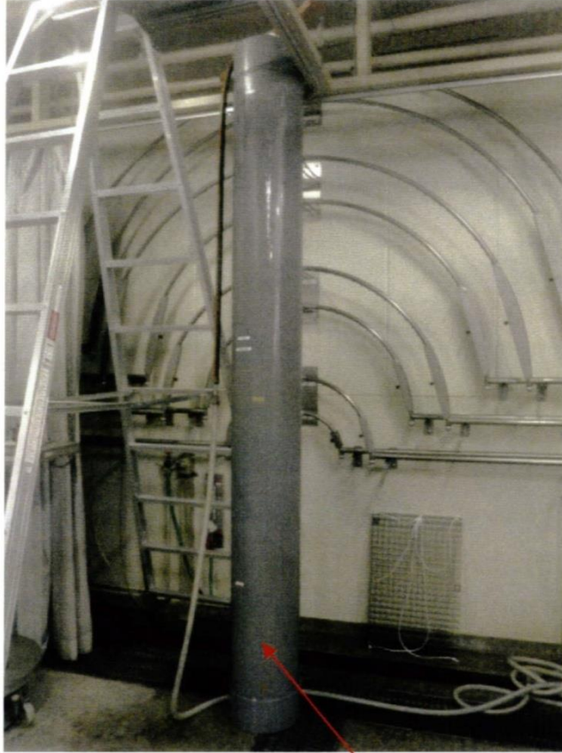
Immersion tank, water-level: 3m
